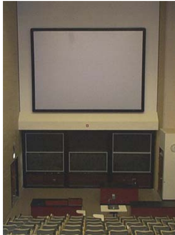
Figure 10. The 13'x18' silvered screen. Note the smudge due to installer's error is visible at top, left-center of the screen.
